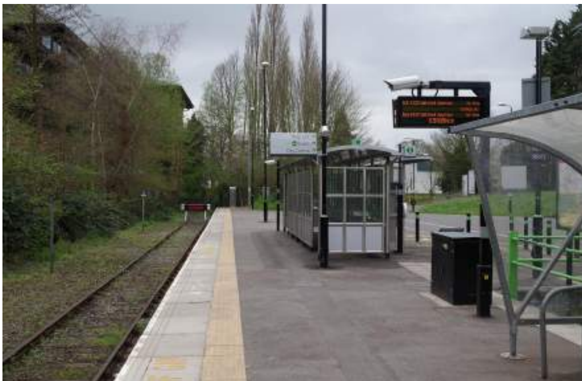
Figure 17 – St Albans Station on the Abbey Line
