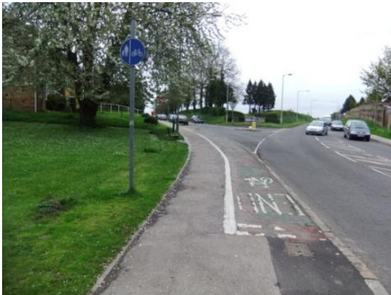
Figure 2 – Termination of cycle track on London Road
